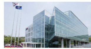
Hydrogen fuel cell R&D center, Korea
